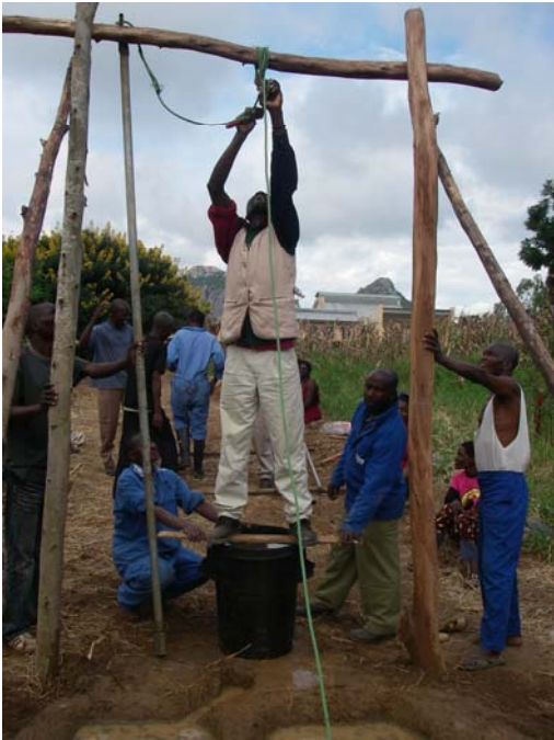
New SWI Team Member, Cornelius Mvula at Well Drilling School
