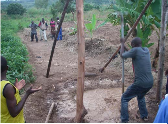
Practice Well with Manual Drilling Rig
